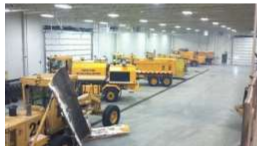
New SRE Building Interior
