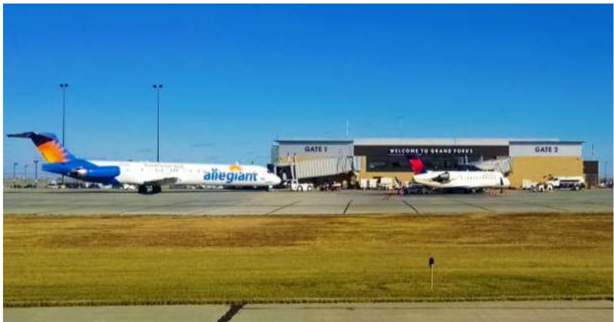
GFK Passenger Terminal & Apron
