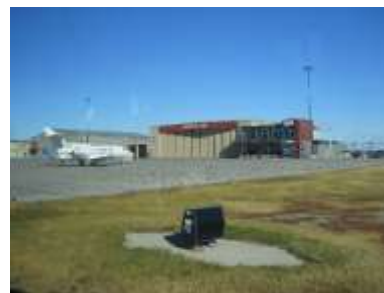
FBO Hangar and Terminal
